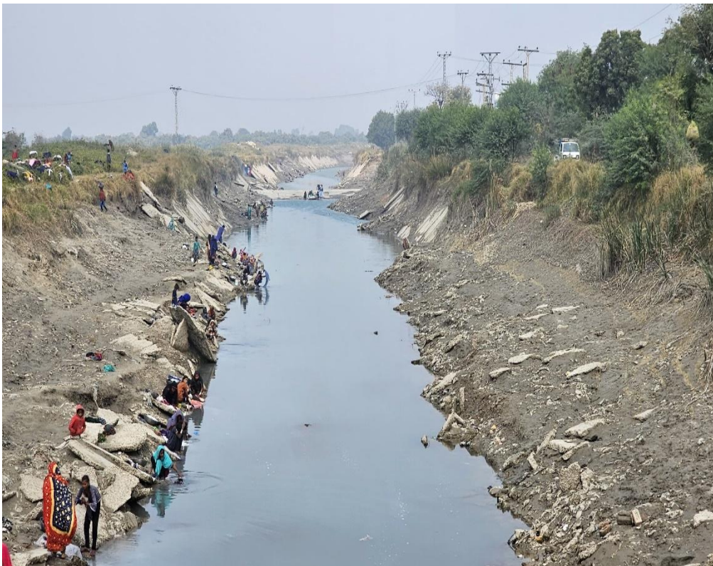
The photograph on the cover page shows the poor condition of the current embankment of Akram Wah Canal.
