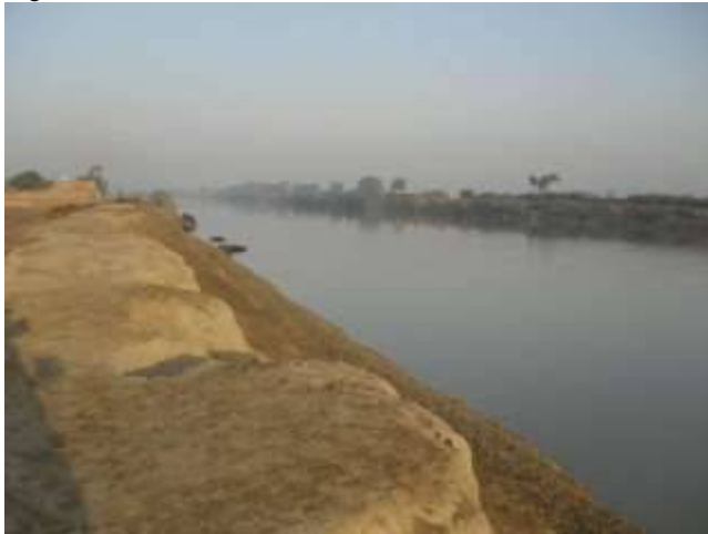
Figure 3.2: Eroded Embankments on the Fulleli Canal
