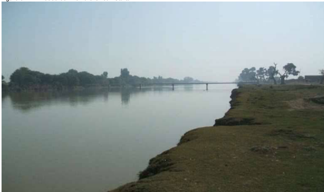
Figure 3.2: Eroded berm on the Ghotki Canal
