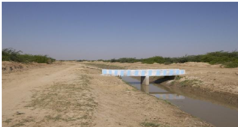
Kandiario minor foot bridge after construction
