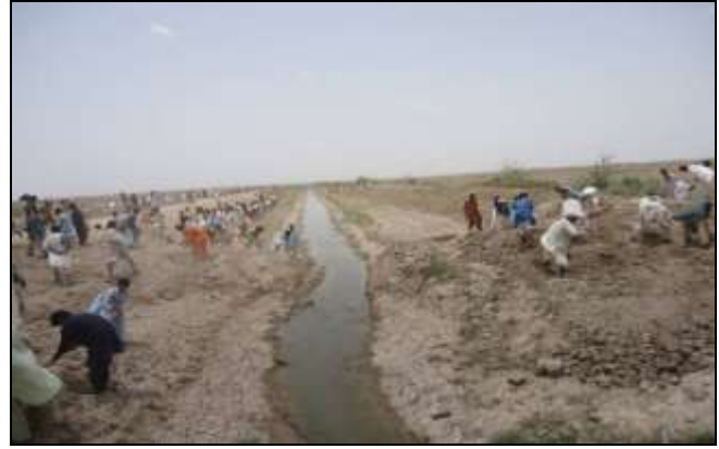
17 L Drain after Rehabilitation Work
