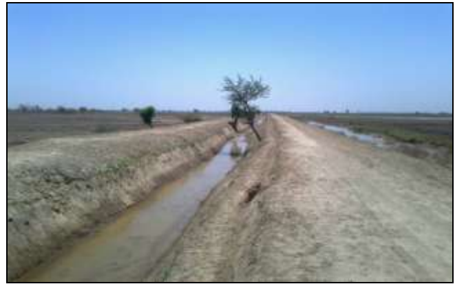
Tegu sur Minor after Rehabilitation Work
