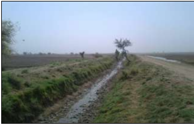
Tegu sur Minor Before Rehabilitation Work
