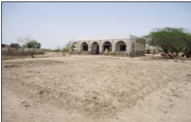
Raised Plate form at GPS Mitho Raiar Umerkot
