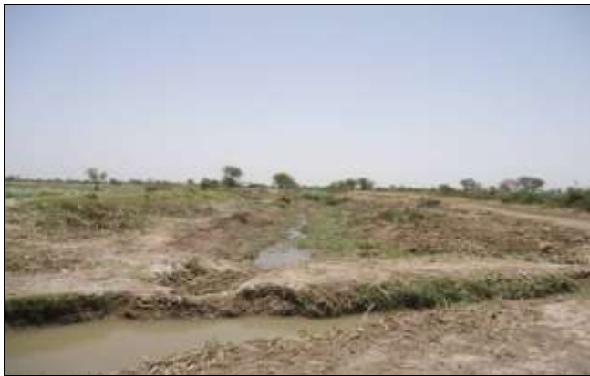
17 L Drain Before Rehabilitation Work
